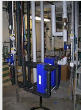
Heat exchangers for district heat and cold supply.
