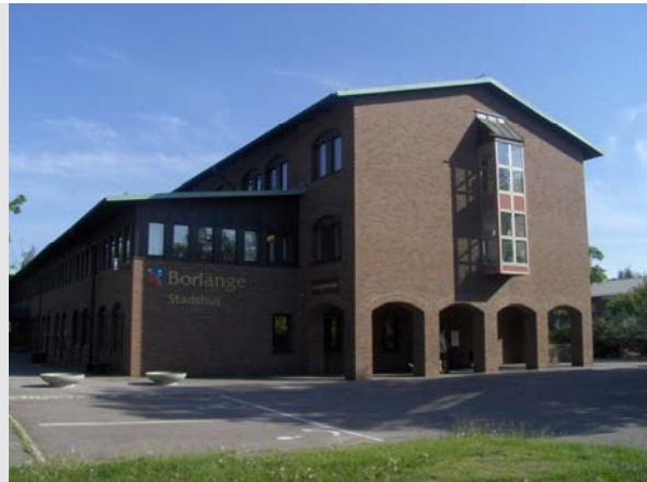
Entrance to the city hall (one of six wings).
